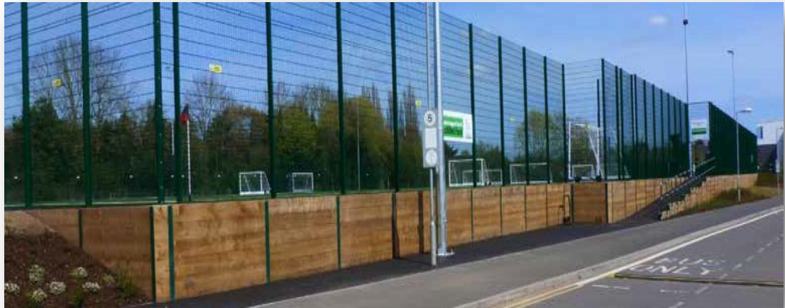
EXAMPLE OF TYPICAL TIMBER SLEEPER RETAINING WALL
